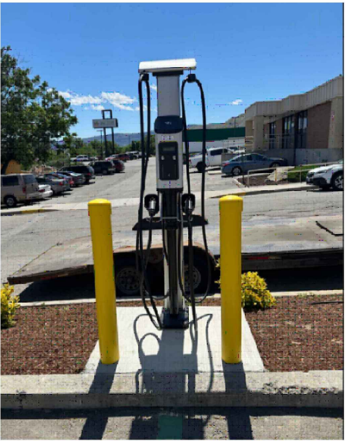
CHARGING STATION WITH CONCRETE PAD - TYPICAL
