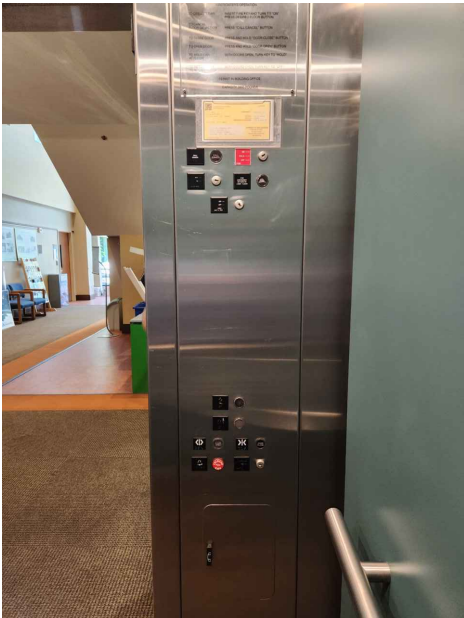
LOBBY ELEVATOR LOWER LEVEL - INSIDE CAR
