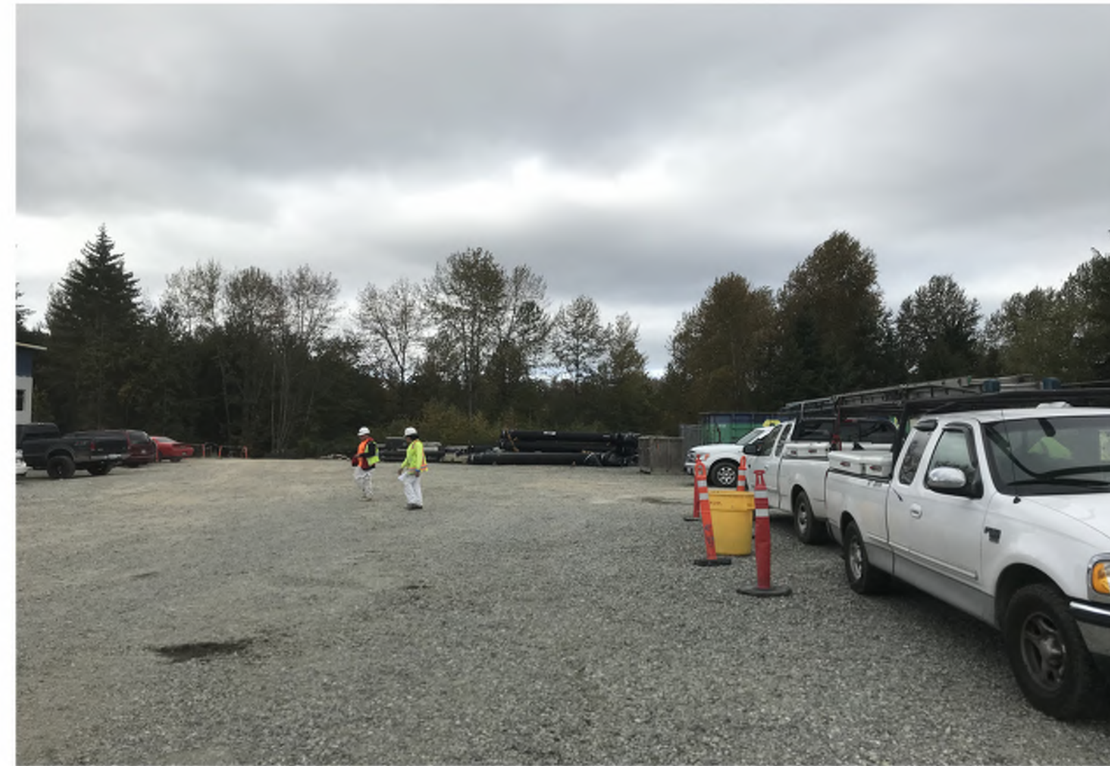
CAMERA 2 - LOOKING WEST FROM INSIDE E. PROP. LINE
