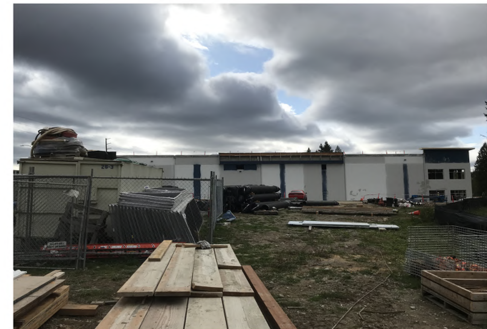
CAMERA 6 - LOOKING SOUTH
