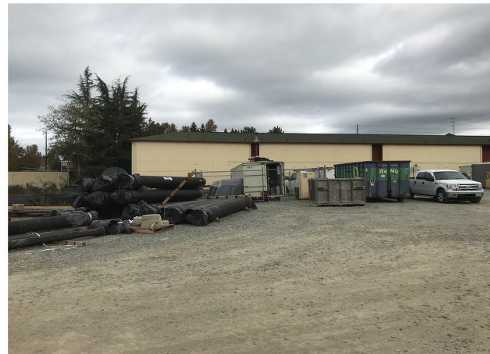
CAMERA 4 - LOOKING NORTH
