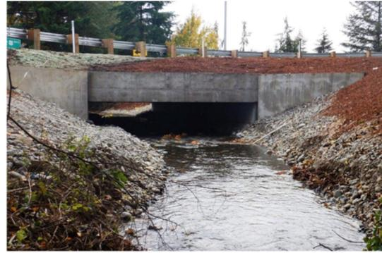
This photo shows an example of a culvert, or a large pipe beneath the roadway, that allows fish passage and reconnects streams.
