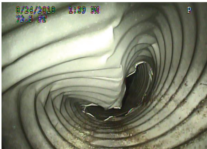
CCTV image of the inside of a damaged corrugated metal pipe.
